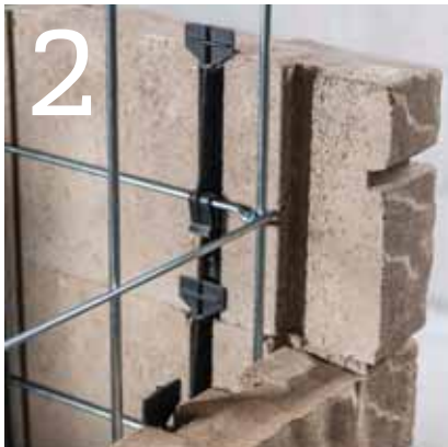
2 Use connector to attach Tandem Veneers to grid
